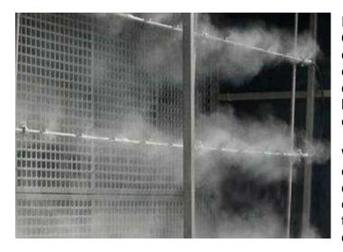
Installing a Harley Humidikool<sup>™</sup> Outdoor Cooling System to aircooled chillers improves the efficiency of their working conditions, as the water mist lowers the temperature of the air entering the condenser.
