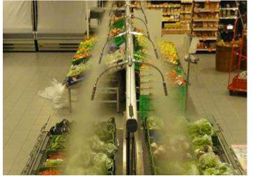
misting system emits a fine water mist on a regular basis. Because of their small size, these water droplets evaporate without becoming wet, preserving the humidity and coolness of the air, preventing dehydration, and maintaining the weight and condition of the goods.
